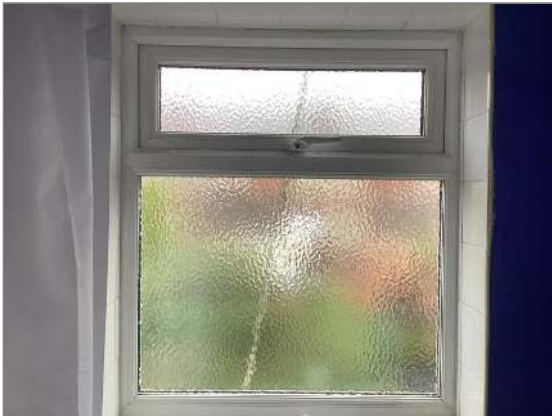
Photo - 50 Bathroom UPVC double glazed window with stiff casement
