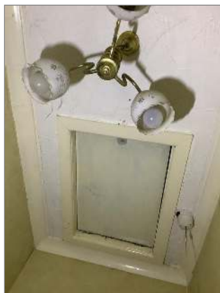
Photo - 84 Textured coating to landing ceiling
