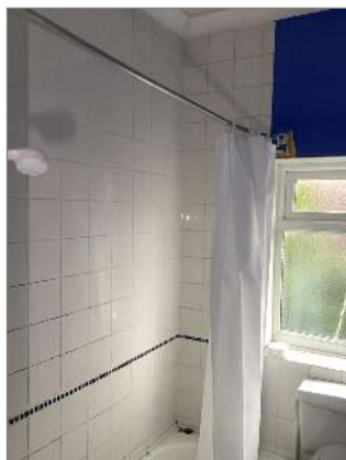
Photo - 99 Ceramic tiles and painted plaster
