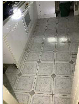
Photo - 123 Ceramic tile to solid floor in kitchen
