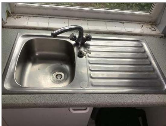
Photo - 142 Brittle sealant to laminate worktop
