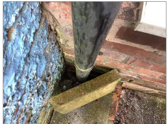
Photo - 21 Downpipe to the rear
