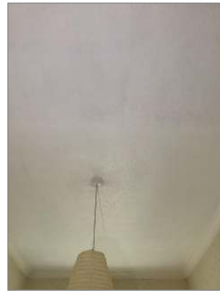
Photo - 81 Wallpaper to rear bedroom
