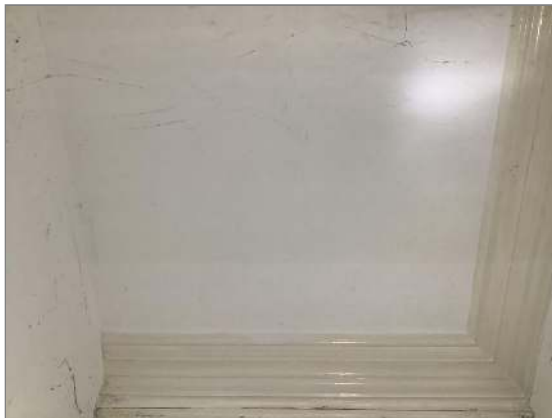
Photo - 88 Wallpaper ceiling to vestibule and front lounge
