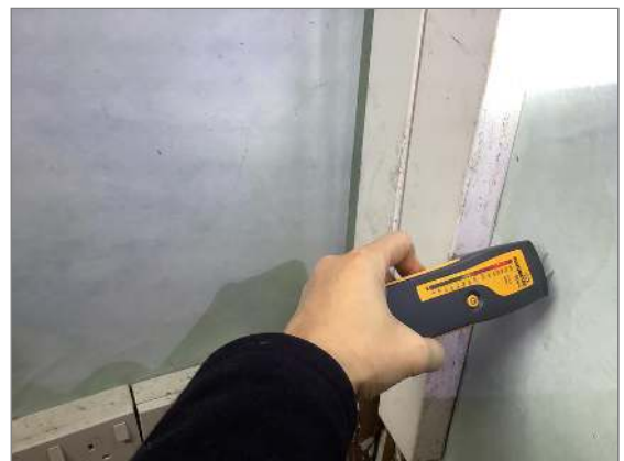
Photo - 112 Chimney breast
