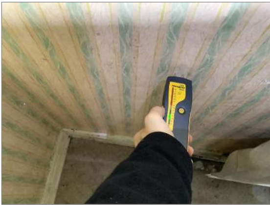
Photo - 95 Front wall
