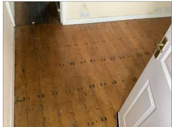
Photo - 121 Timber floorboard to front lounge
