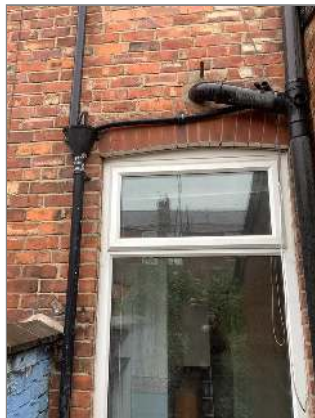
Photo - 20 Downpipe to the rear
