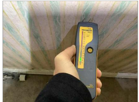
Photo - 94 Front wall
