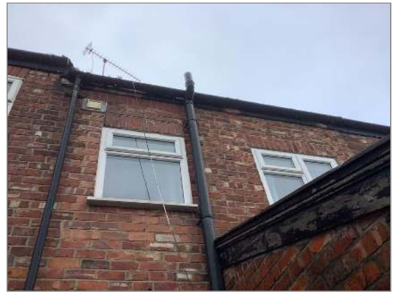
Photo - 19 Rainwater goods to the rear
