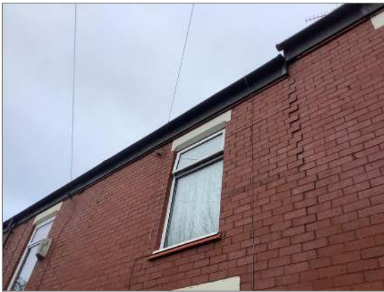
Photo - 18 Rainwater goods to the front
