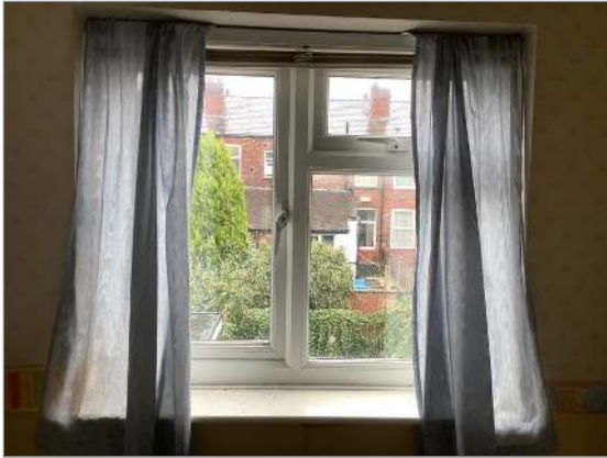
Photo - 48 Rear bedroom UPVC double glazed escape window
